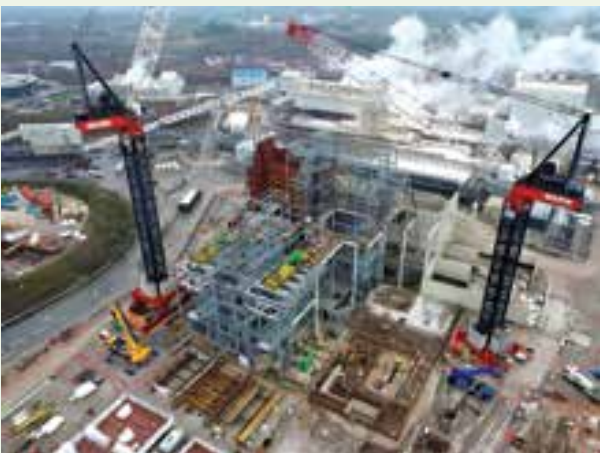
Favco Tower Cranes for Lstock Sustainable Energy Plant, Cheshire, United Kingdom
