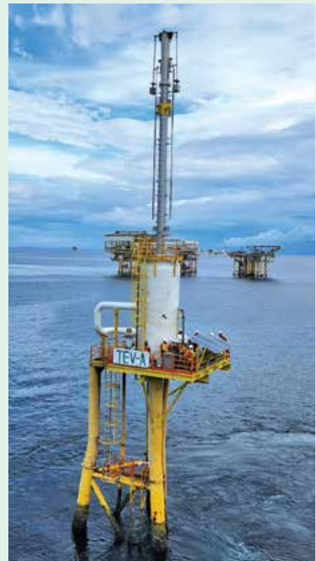
Advanced Flare System Installed and Commissioned to meet zero continuous venting directives for Petronas Carigali in Bintulu offshore, Sarawak by Exact Automation
