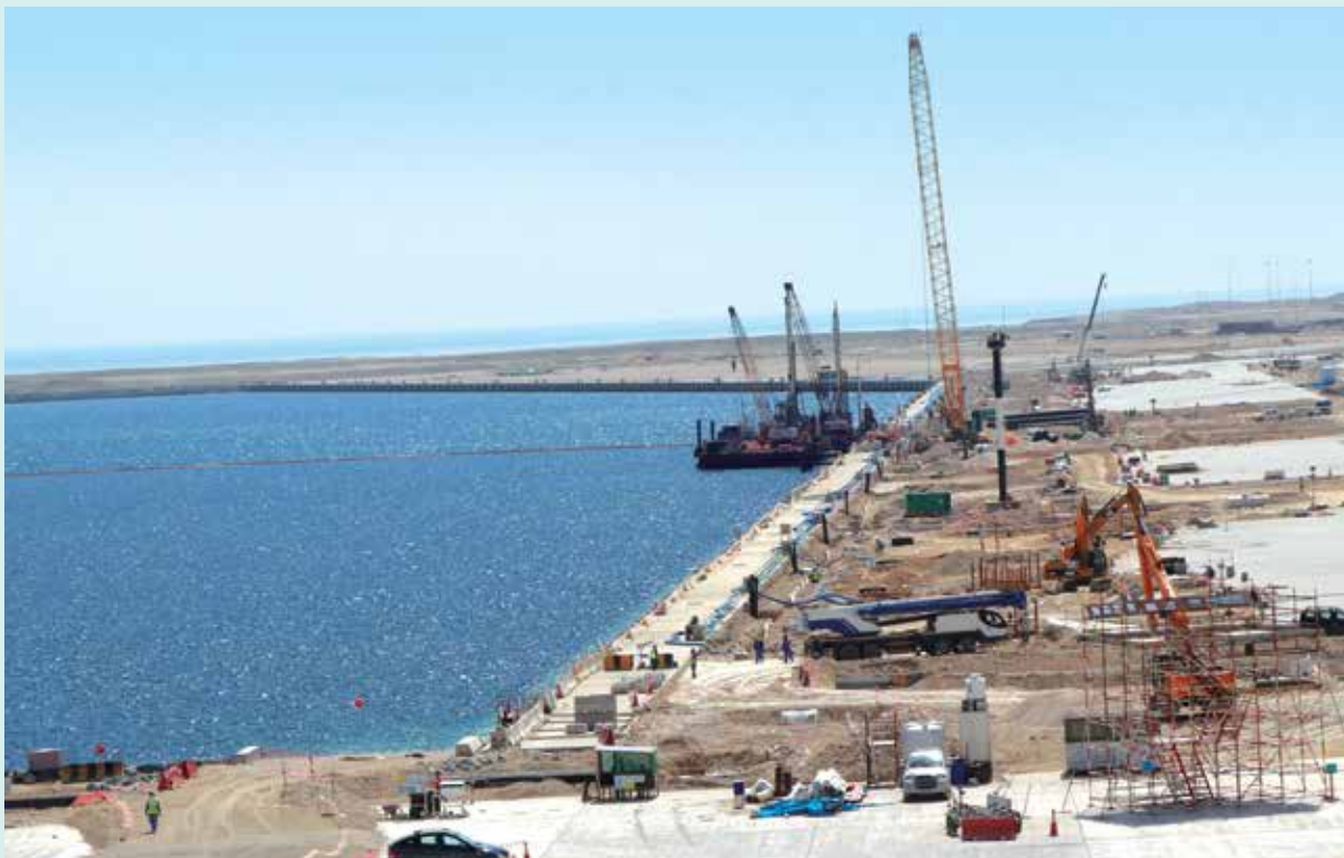
Syncrolift Project - Piling, Basin Water Depending & Slipway Construction, Qatar
