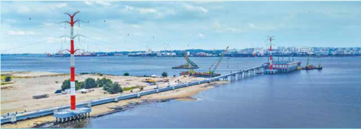
Construction of Jetty and Platform for Senibong Switching Station and Overhead Line from PMU Senibong to Switching Yard Station at Senibong, Johor Bahru
