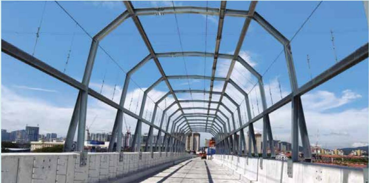
Noise Barrier Enclosures Over High Tension Cable Crossing for KVMRT Line 2
