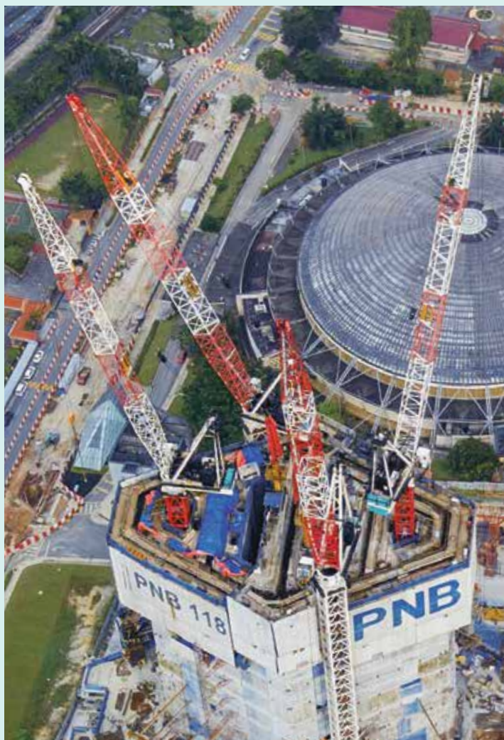
Favelle Favco - Tower Crane for Construction of PNB's KL 118, Malaysia
