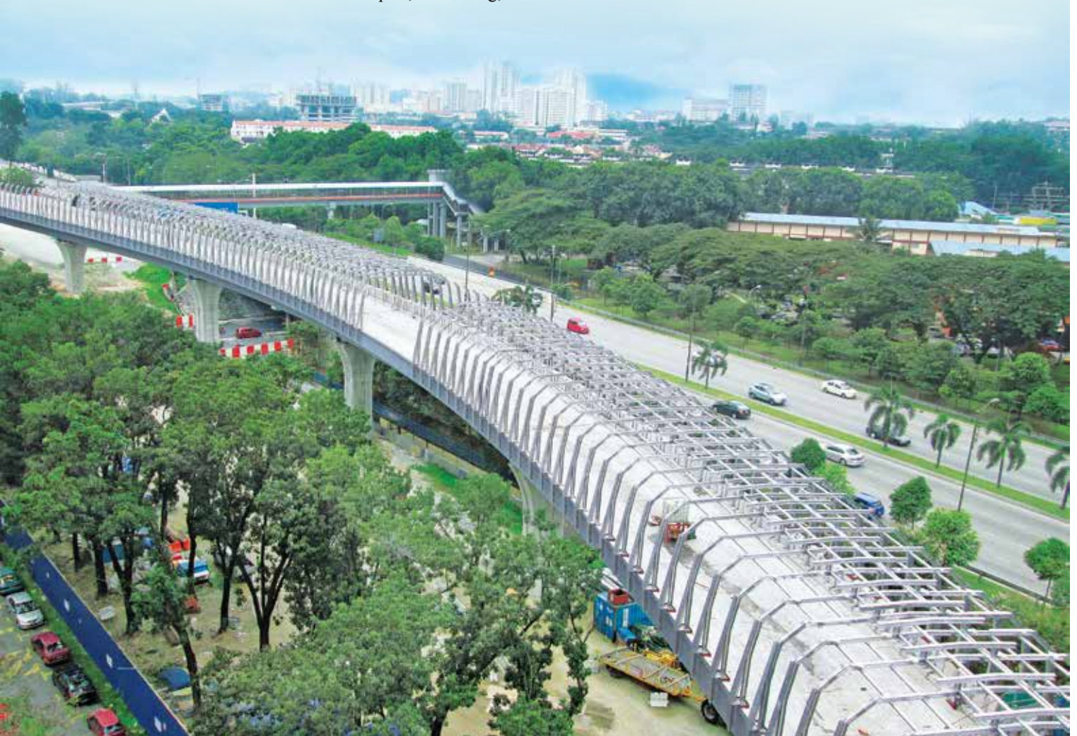
Klang Valley Mass Rapid Transit (“MRT”) Jajaran Sg. Buluh to Kajang - Full Enclosure Noise Barrier Structure
