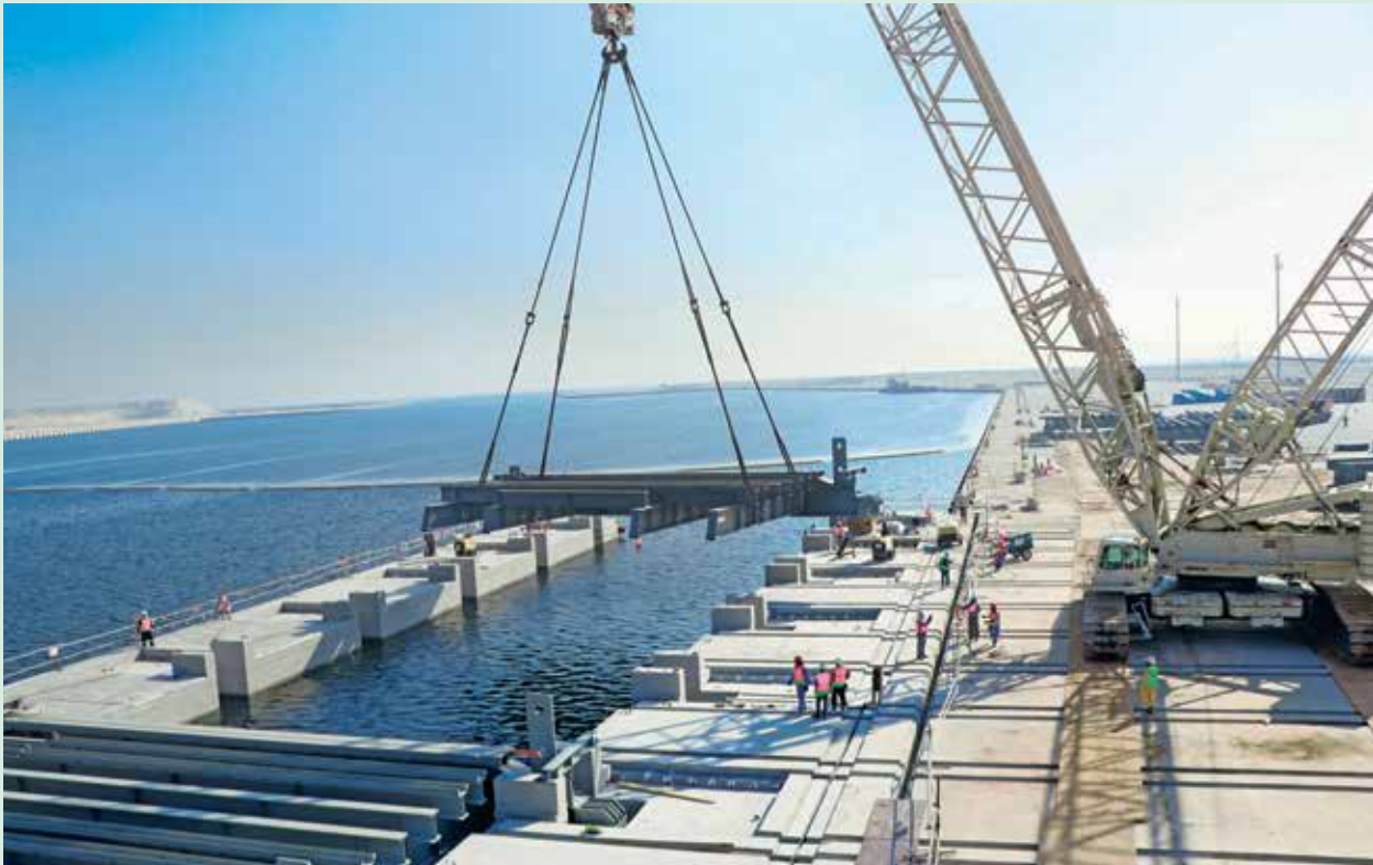
Installation of Shiplift Platform in UM ALHOUL ECONOMIC ZONE, QATAR
