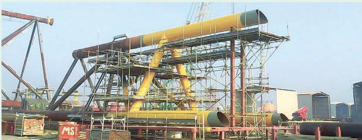
Fabrication of Offshore Jacket for Central Processing Platform for Tembakai (Oil) Development, Offshore Terengganu, Malaysia
