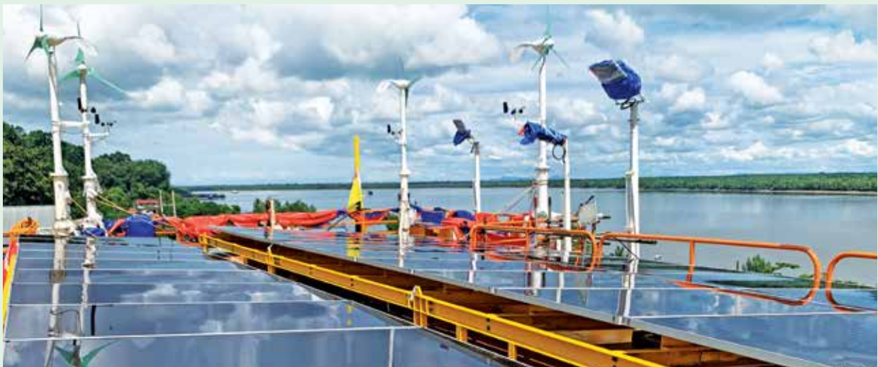
Solar and Wind Hybrid Renewable Power System, TIMI Gas Field, Malaysia by Intelligent Automation Division
